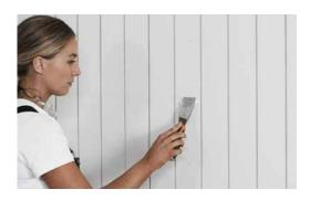
• Use putty to fill in any nail or screw holes, allow adequate drying time before you sand and paint.
