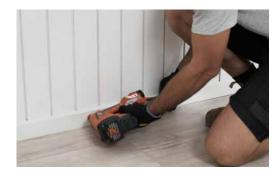
· Lastly, install skirting boards, cornices and dado rails as necessary.
