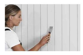
• Use putty to fill in any nail or screw holes, allow adequate drying time before you sand and paint.
